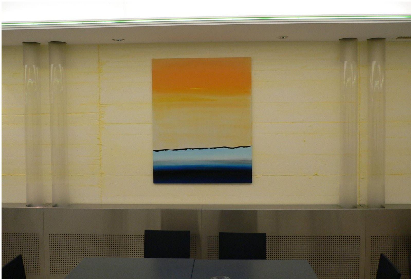
Pictures framed by air conditioning conducts in glass- and stainless-steel
